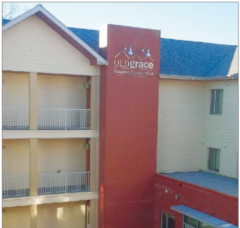
FIGURE 1: False chimney at the Old Grace Housing Cooperative. Note that the chimney is the large red rectangular structure in the centre of the photograph. Photo credit: Ken De Smet, Manitoba Government.
