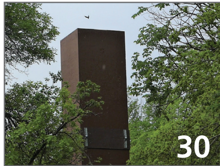
30 Previous attempts to provide purpose-built artificial chimneys in Manitoba for the threatened Chimney Swift have not attracted swifts. A new design of artificial chimney was constructed in Winnipeg and moved to the Assiniboine Park Zoo. Chimney Swifts bred in this tower during the summer of 2019, the first confirmed use of purpose-built artificial habitat in western Canada.
