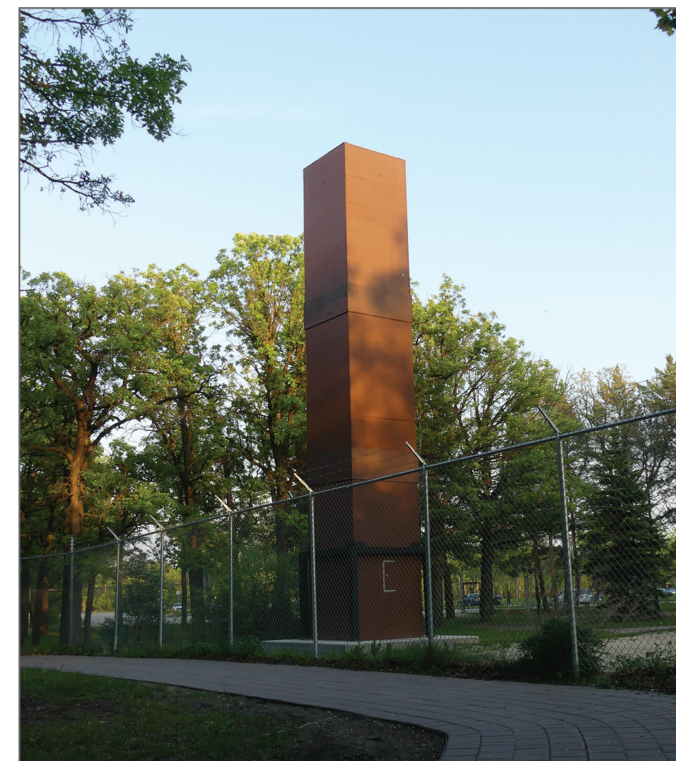
FIGURE 1. The tower in its current location at Assiniboine Park Zoo. Note the three distinct sections, the supportive bracket around the base and the concrete pad. Photo credit: T. Poole.
