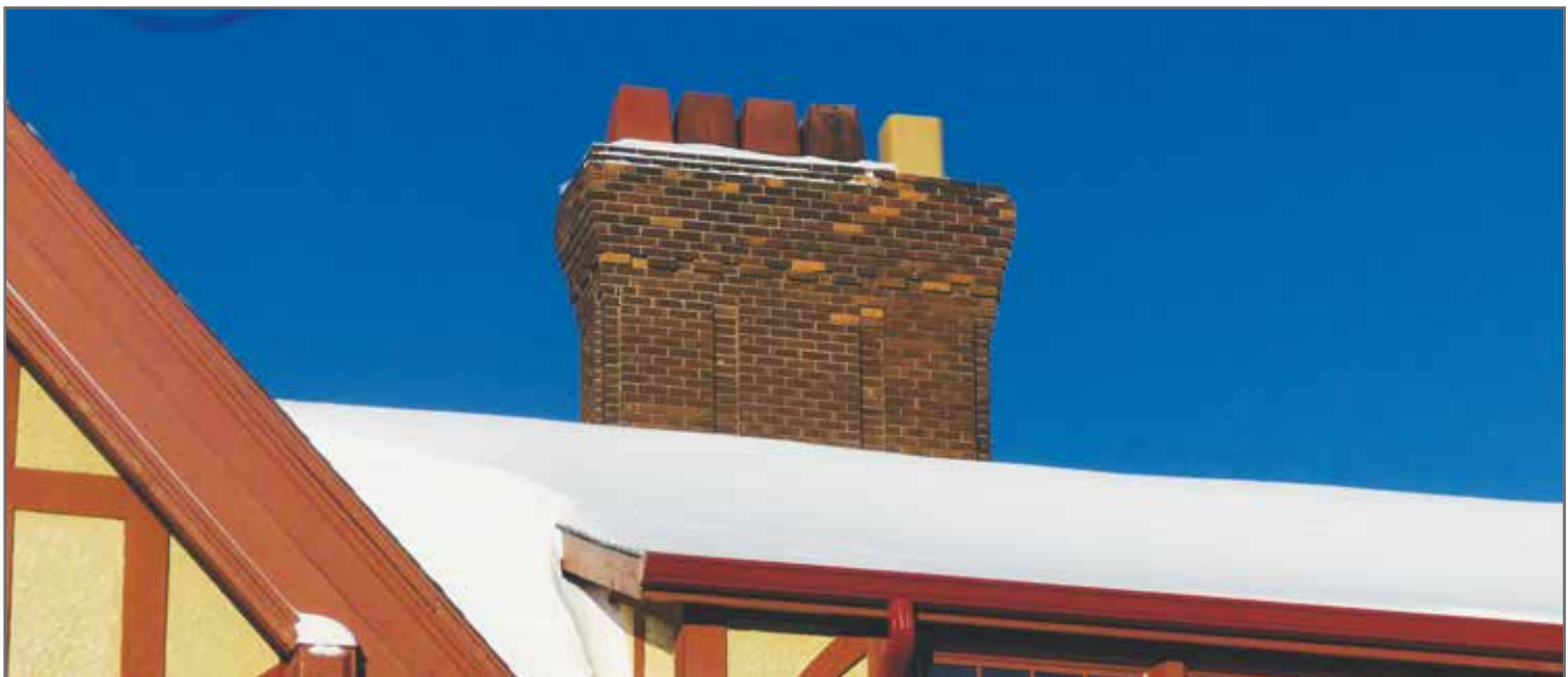
FIGURE 5. Chimney at the Granite Curling Club with multiple clay pots. Photo credit: Timothy Poole.
