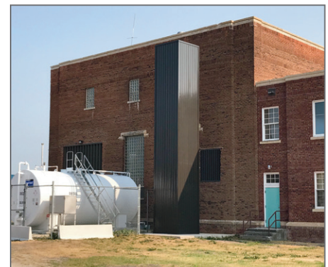
FIGURE 3: Tower T4 at the Selkirk Mental Health Centre. Photo credit: Robert Stewart.
