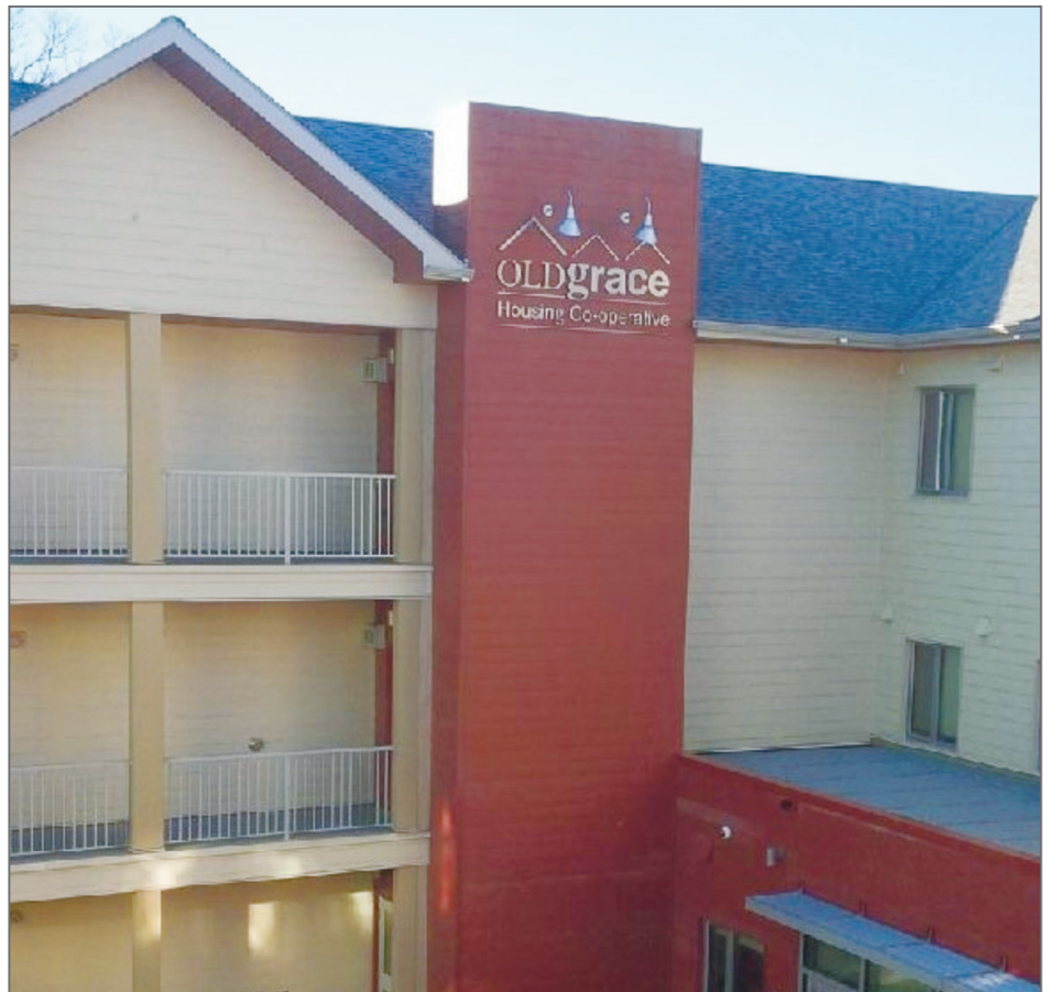
FIGURE 1: False chimney at the Old Grace Housing Cooperative. Note that the chimney is the large red rectangular structure in the centre of the photograph. Photo credit: Ken De Smet, Manitoba Government.
