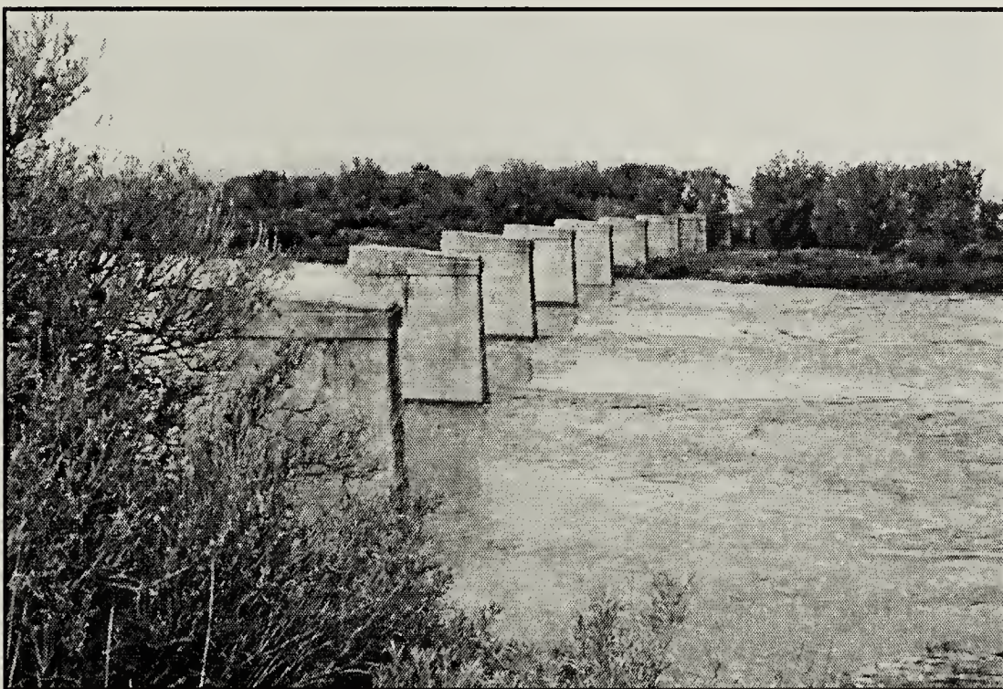
Figure 1. Pillars of the railroad bridge, June 11, 2005
