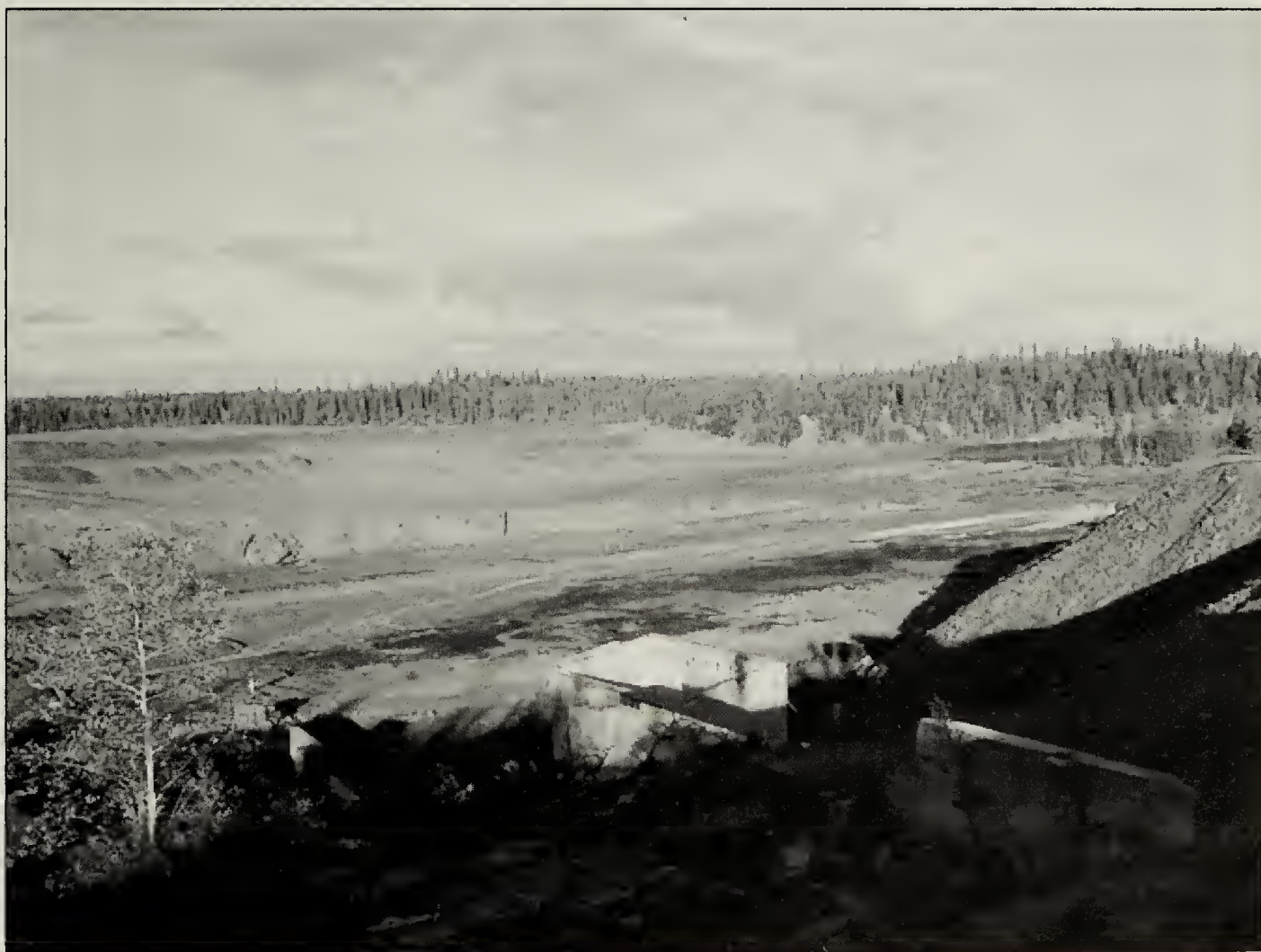
Figure 1. Sherritt-Gordon mine tailings pile, July 2005. The runoff from the pile collects on the right before it enters Camp Lake.
