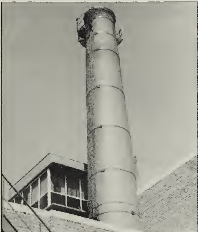
Figure 3. Nest of raven on metal walkway near top of a 37m tall chimney at Deer Lodge Centre, Winnipeg, 22 May 2006
