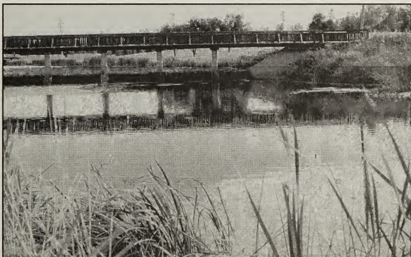
Figure 3. South footbridge and weir
