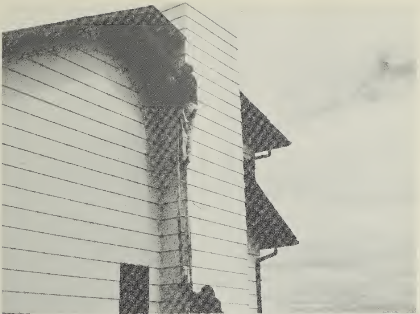
Figure 4. Owl nest on sloping lower roof segment (opposite Houston's head) on temporarily unoccupied Polsom house, north of Dilke, 13 May 1989 Kelly Wylie
