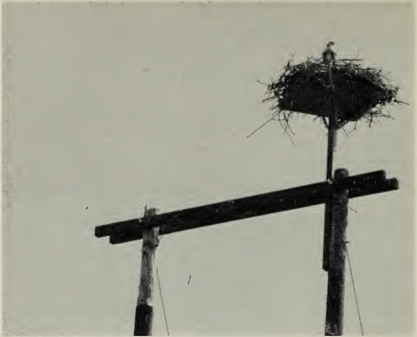
New location of Osprey nest on structure above live power lines.
