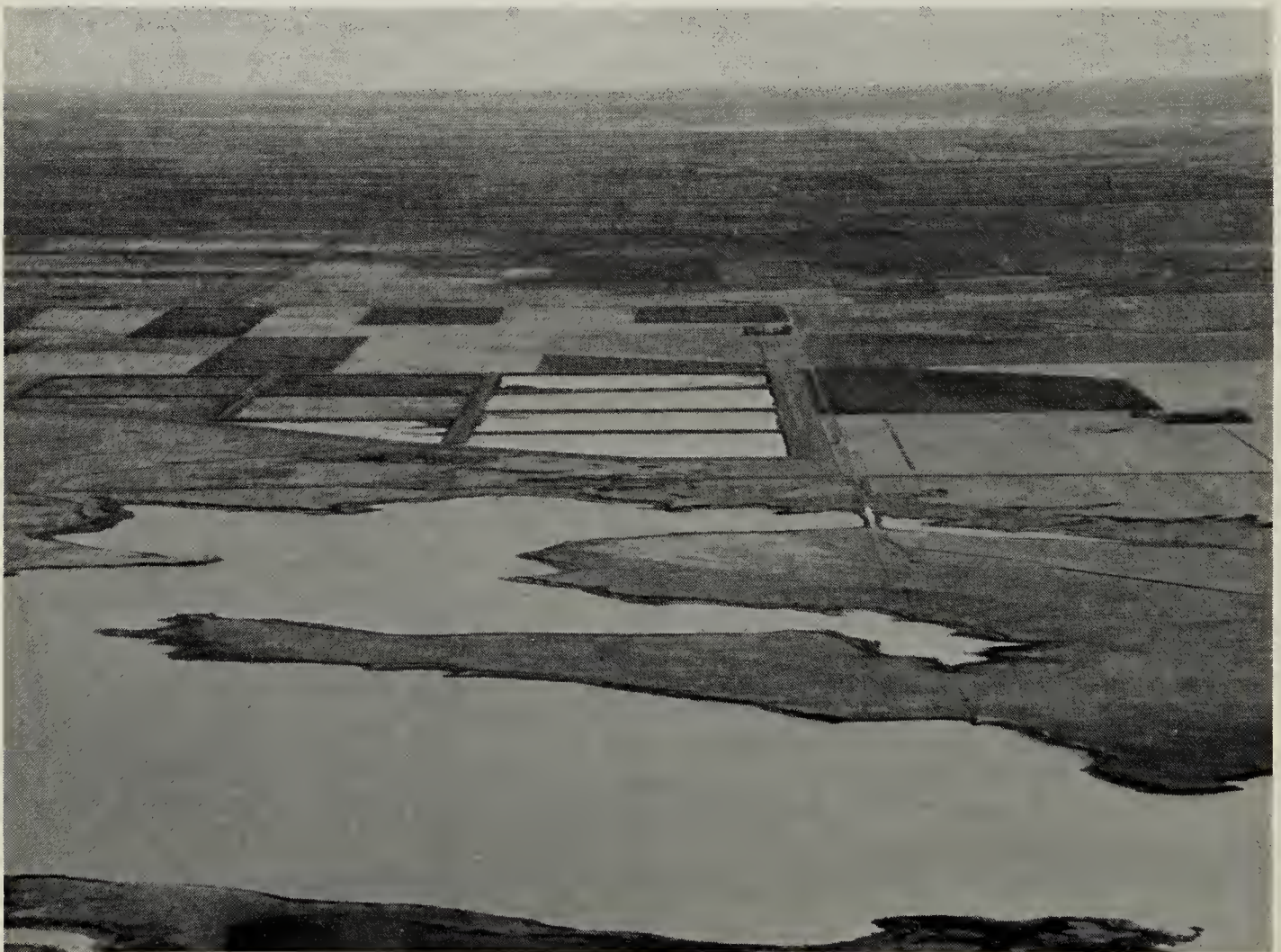
Figure 1. Aerial view of the nine lagoon cells.
