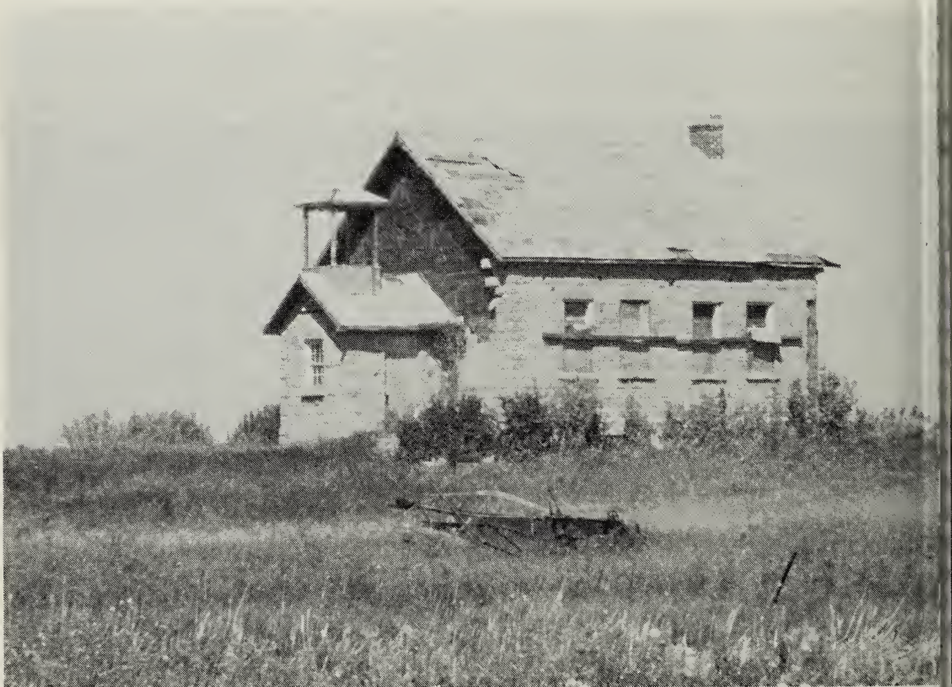
Old school north of Maryfield, Saskatchewan. Abandoned building sites often vegetated with Smooth Brome, which moves outwards from these sites.
