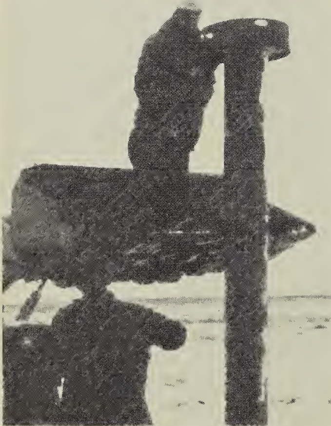
Fig. 3 Placing of unsuccessful oil drum platform. C. S. Houston
