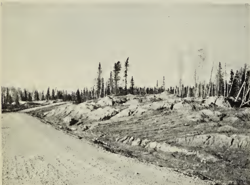
Fig. 7. Erosion along the present road to Besnard Lake is particularly severe where the road crosses the Montreal River. As a result of this erosion the Montreal River in spring changes from a clear stream above the road to a brown turbid stream below it. Such increased turbidity in a spawning area during the critical time of spring runoff may have a drastic effect on spawning fish.
