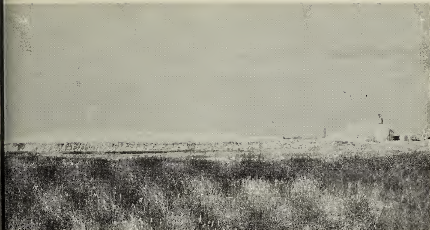
The Chaplin Lake processing plant and sodium sulphate stockpiles.
