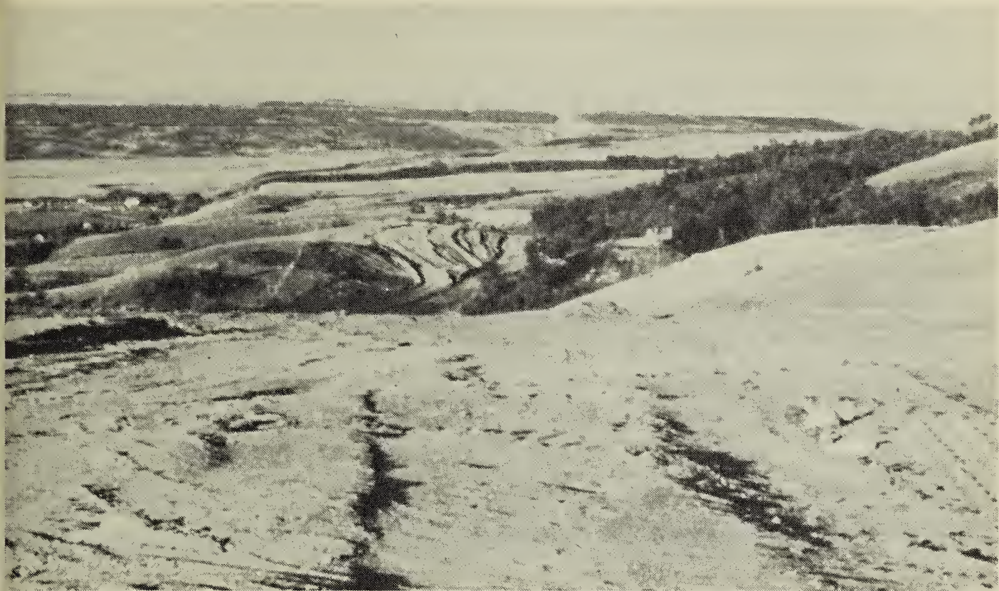
Construction of #6 Highway across the Qu'Appelle Valley
