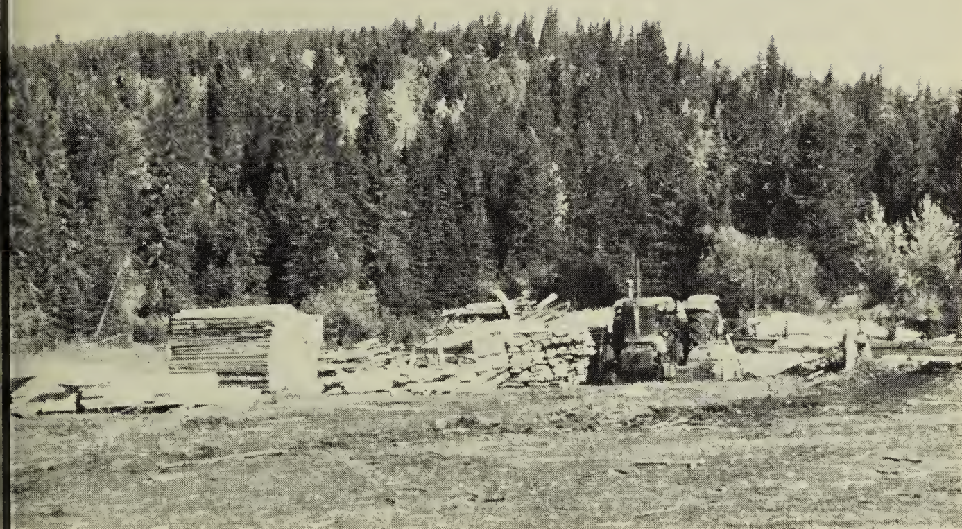
Sawmill operation along Mink Creek, West Block
