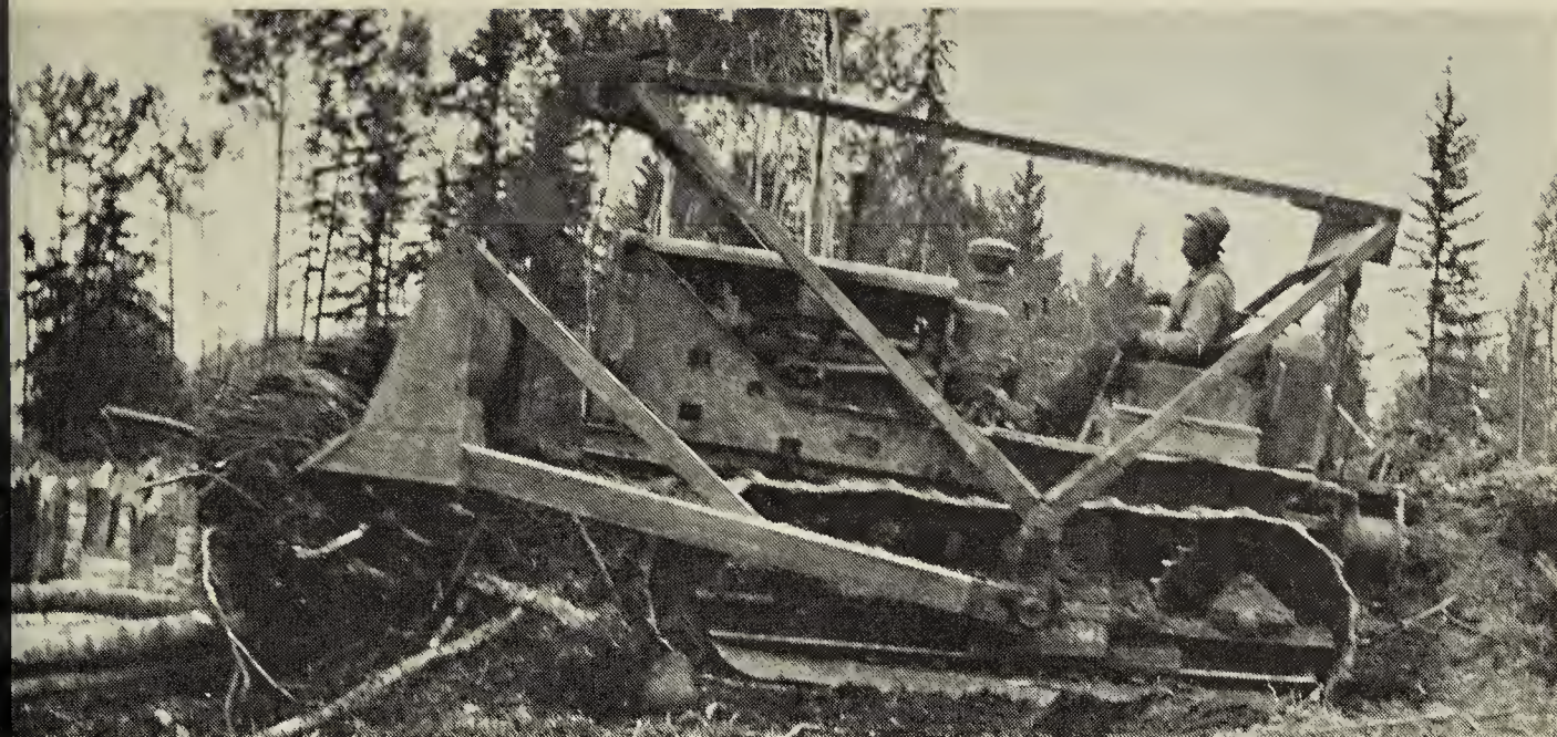
Clearing stumps by bulldozer
