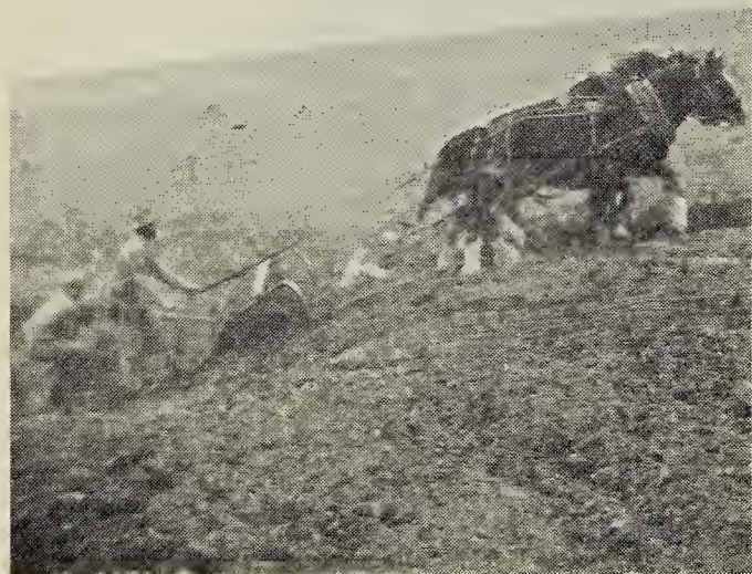
Team work — Steve Mann and his son Robert building an earthwork dam to hold water for livestock and garden.
