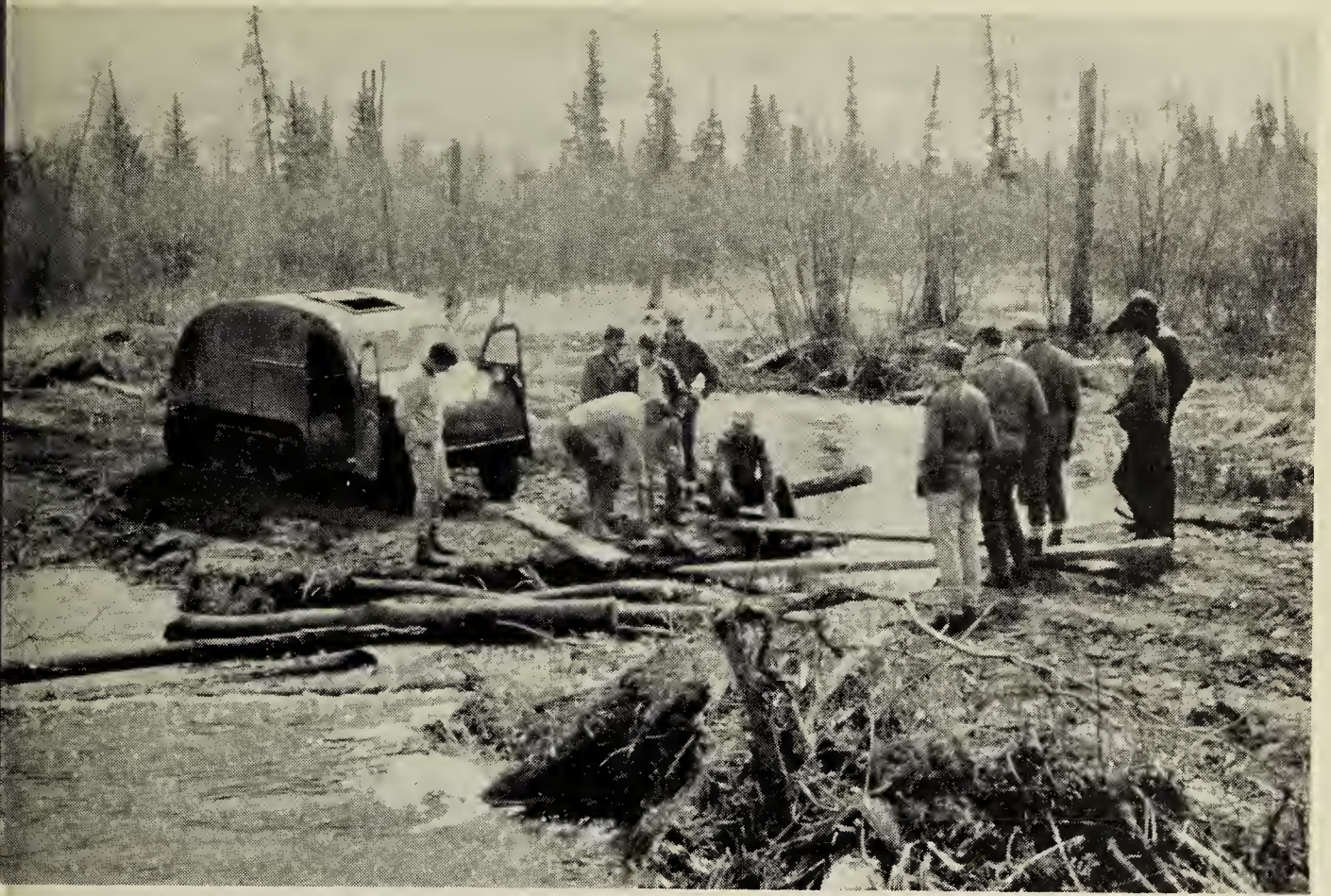
Preparing to cross a spring washout
