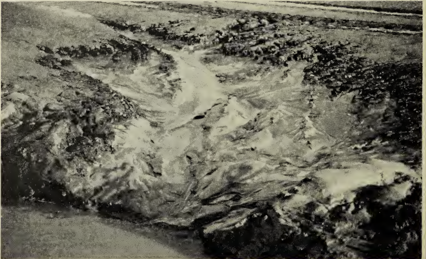
Erosion below a bull-dozer track
